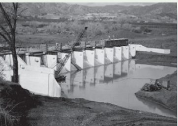
Courtesy Solano County Water Agency, Photography by E.S. Ensor Putah Creek Diversion Dam spillway under construction
